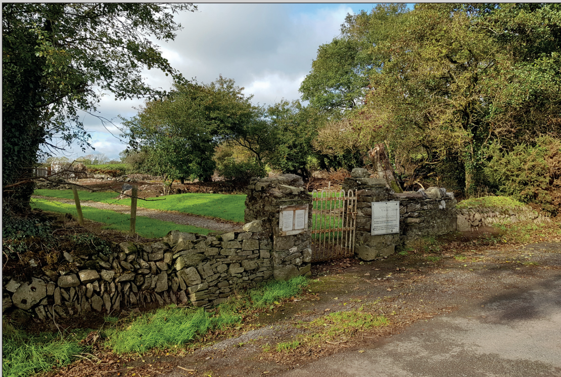
Field walkover survey, ruined church and churchyard at Ballyspillane West - (RMP CO065-083002-)
